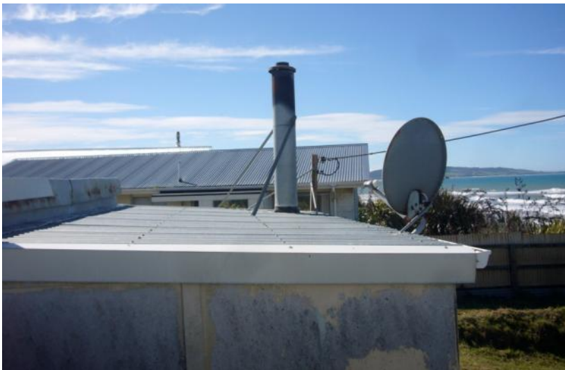
Figure 99. View north over lean to kitchen roof, GB March 2014
