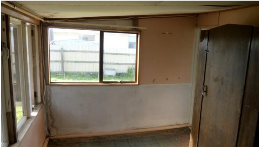
Figure 182. North wall of bedroom, GB March 2014
