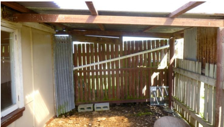
Figure 86. South wall of lean to carport GB March 2014
