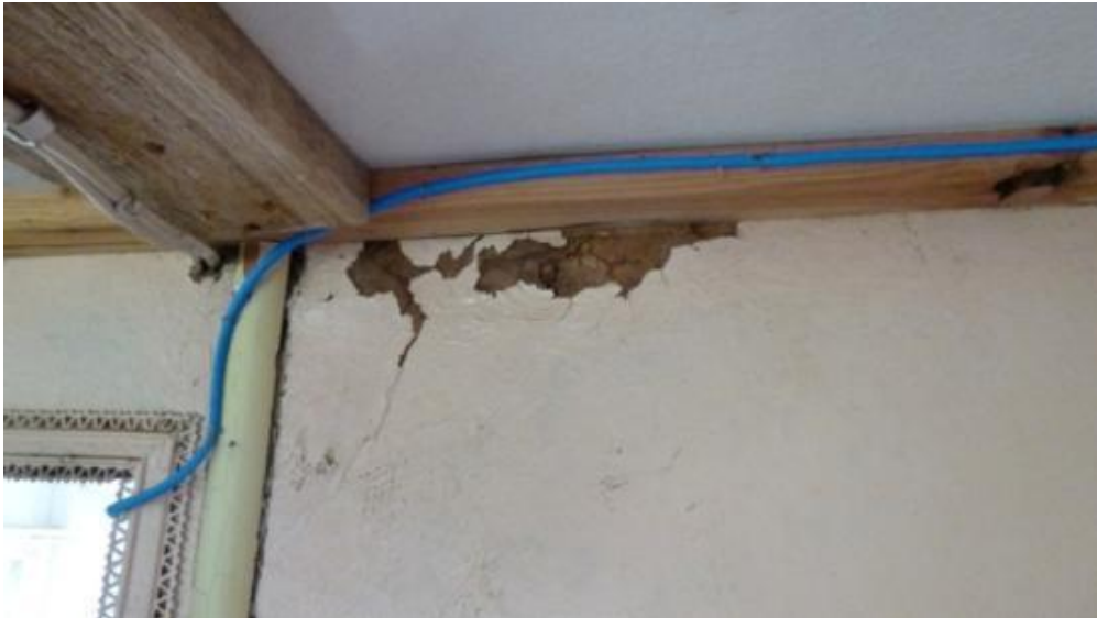
Figure 144. Ceiling in bedroom, east wall, GB March 2014
