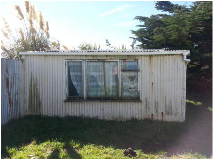
Figure 148. South elevation of the shed, LK March 2014
