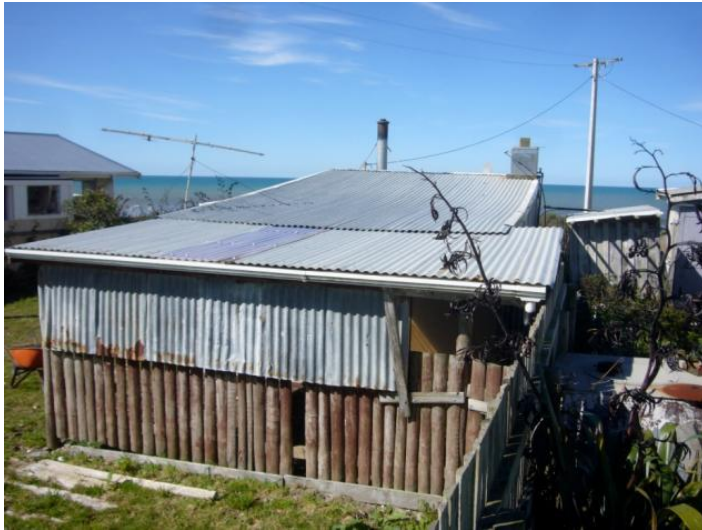
Figure 171. View east over roof of the crib and carport lean to, GB March 2014
