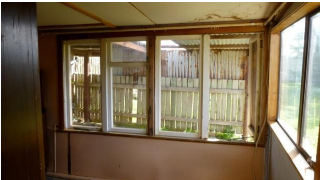
Figure 135. West wall of bedroom, GB March 2014
