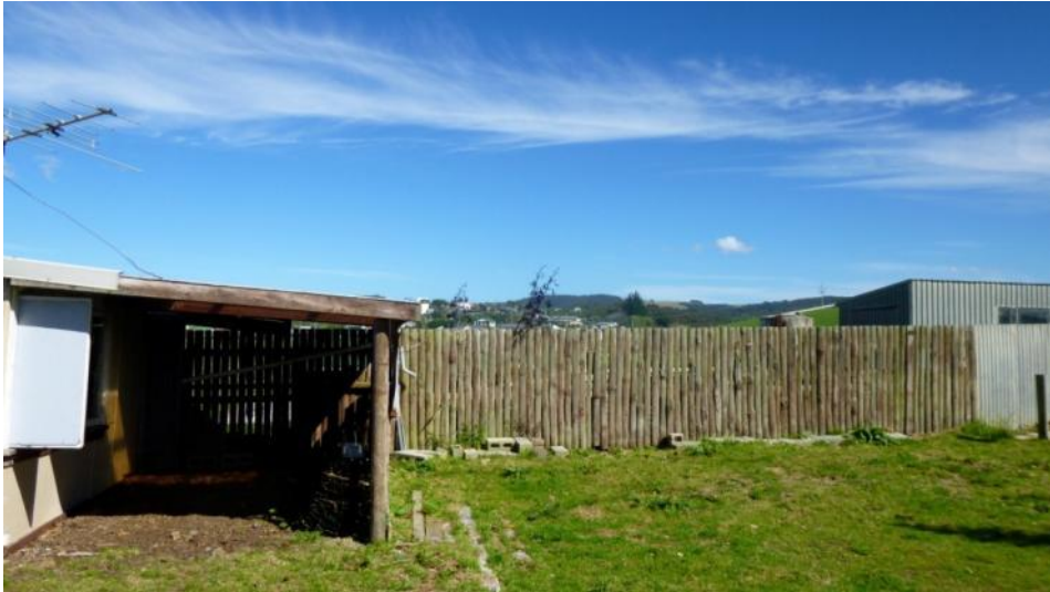
Figure 85. North elevation of lean to carport showing south boundary fence GB March 2014
