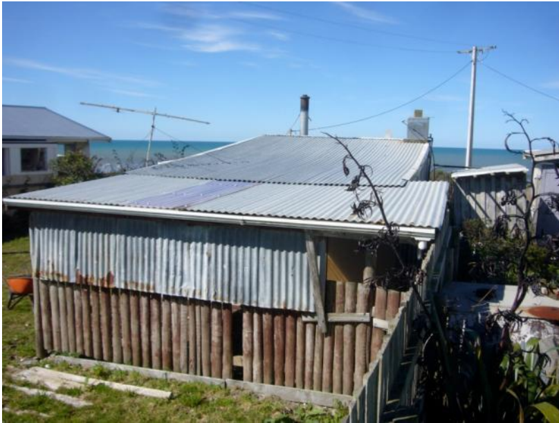
Figure 98. View east over roof of the crib and carport lean to, GB March 2014
