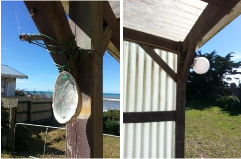
Figure 83. Paua shell on porch post (left) Figure 84. Porch wall detail (right) GB March 2014
