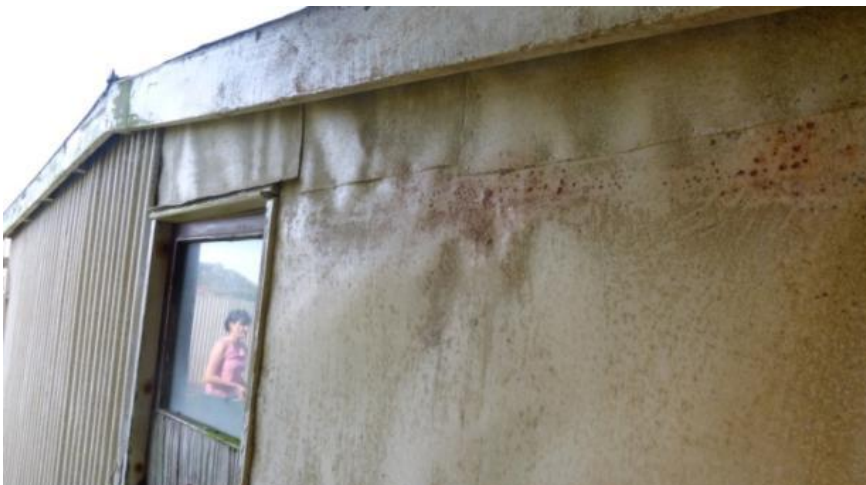
Figure 149. East wall showing material junctions, LK March 2014
