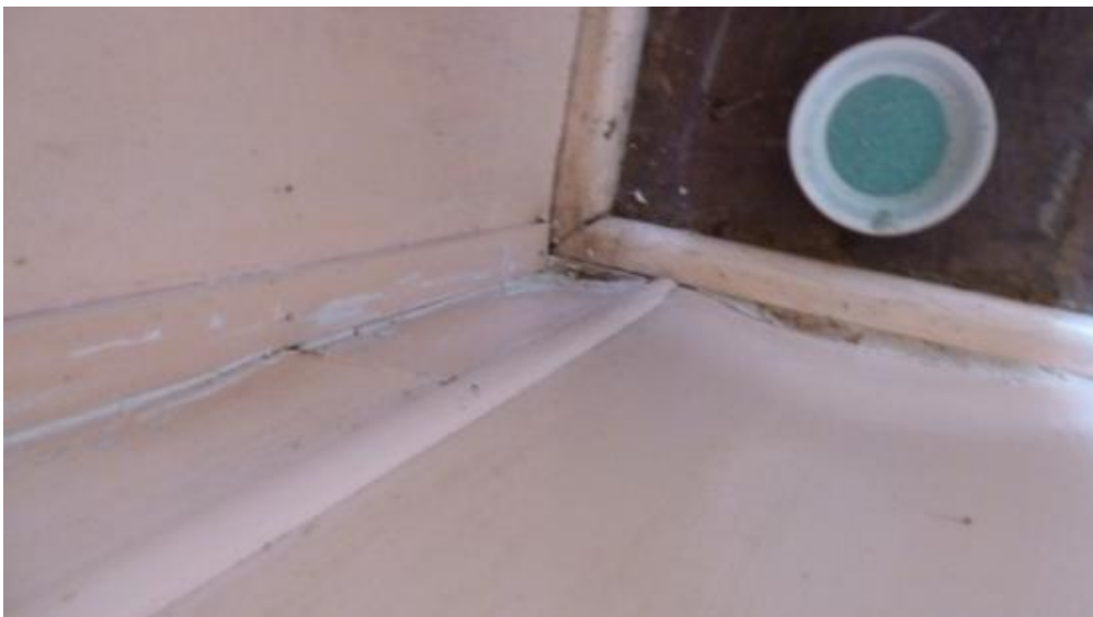
Figure 146. Floor / wall south west corner, GB March 2014
