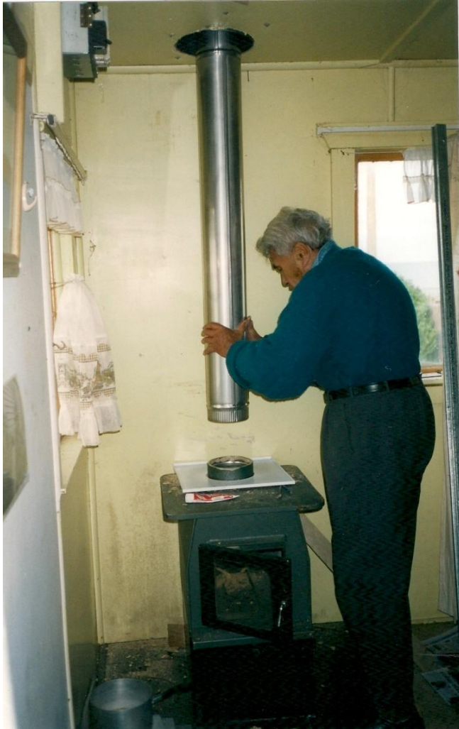
Figure 50. Hone fitting the flue, 2002. Photograph: Jeremy Hay
