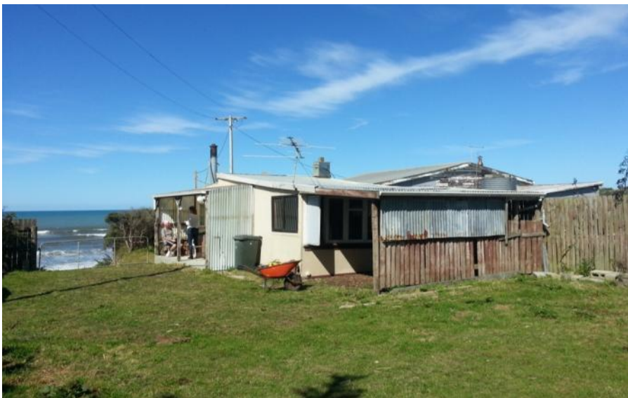
Figure 71. North West corner of the crib. Photograph: LK March 2014.
