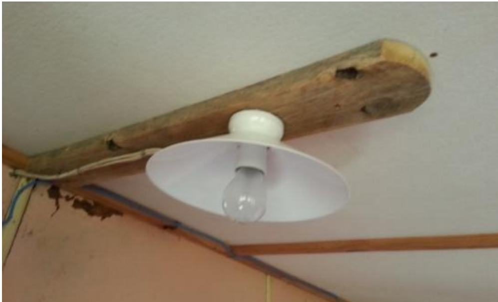
Figure 145. Light fitting in bedroom, GB March 2014
