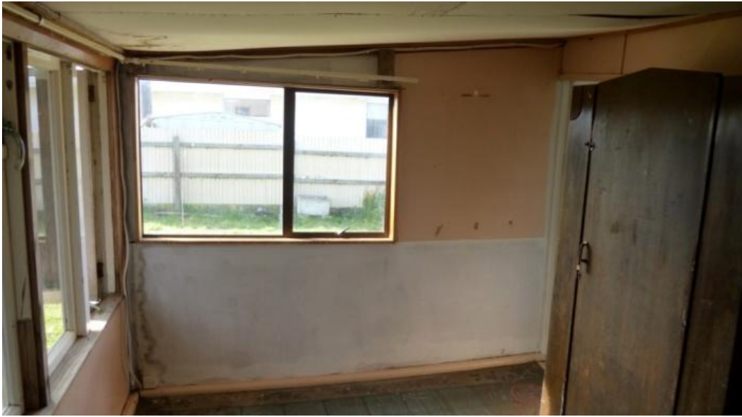
Figure 133. North wall of bedroom, GB March 2014
