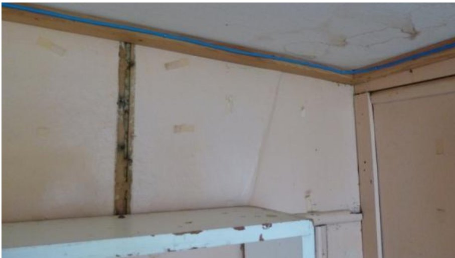
Figure 139. South west corner bedroom ceiling, GB March 2014
