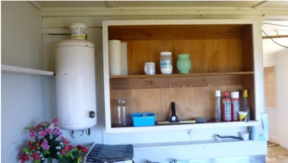
Figure 128. Kitchen cabinetry and boiler unit on west wall of kitchen, LK March 2014
