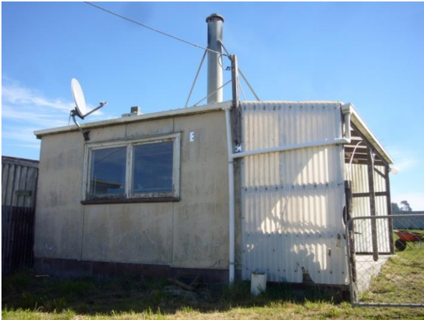
Figure 161. East Elevation of the crib, LK March 2014
