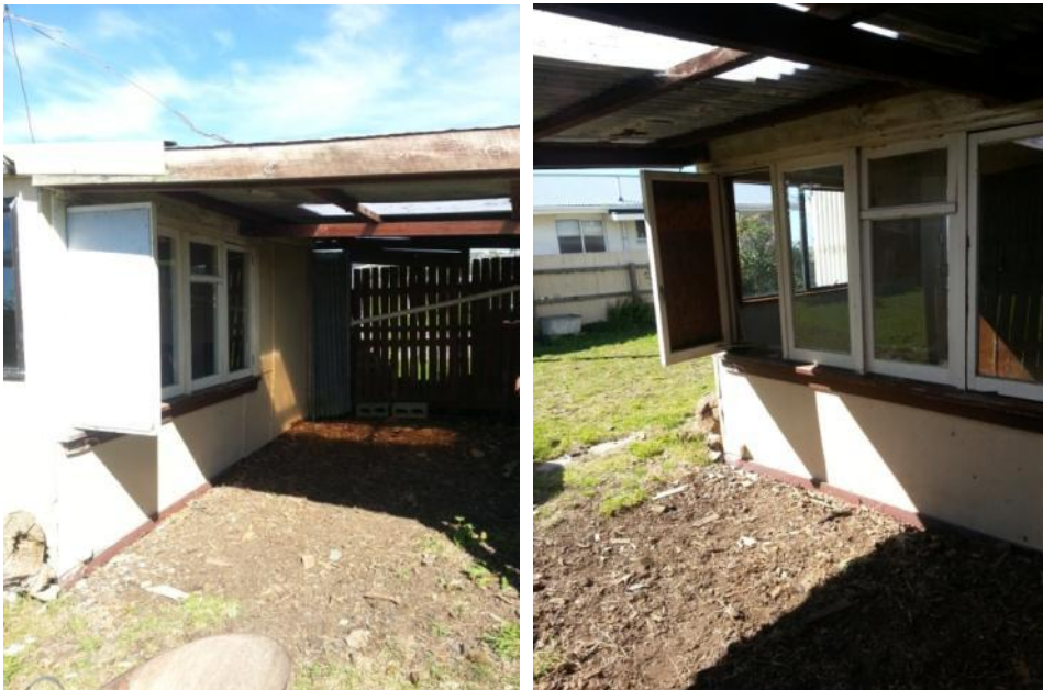
Figure 89. West wall of crib, showing bedroom windows, GB March 2014
