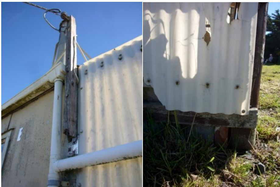
Figure 74. Power line detail (left) Terrace edge (right) Photographs: LK March 2014.
