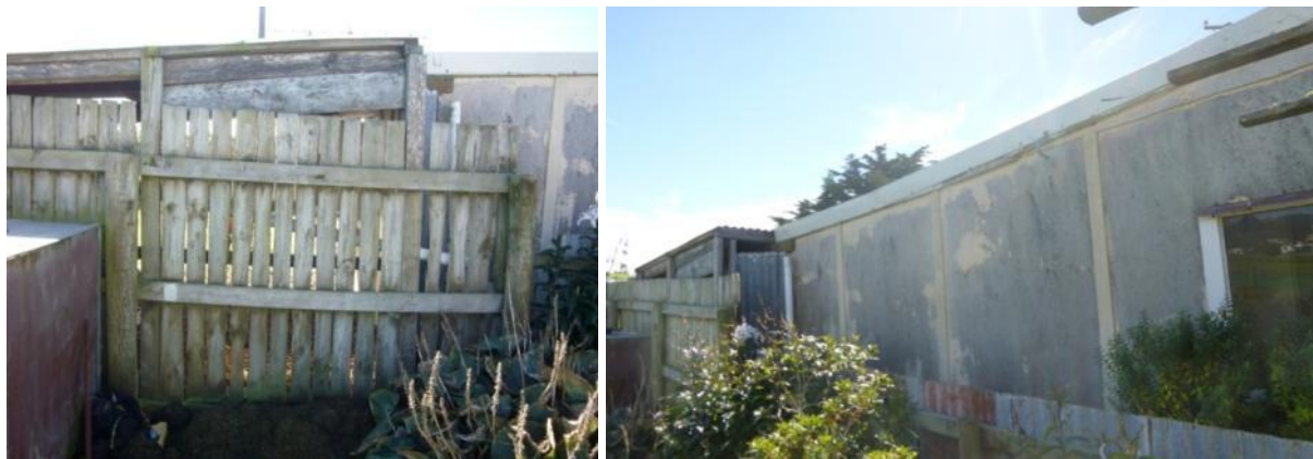
Figure 169. South wall of lean to carport (left) Figure 170. South wall of crib. view from neighbouring property looking west. LK March 2014
