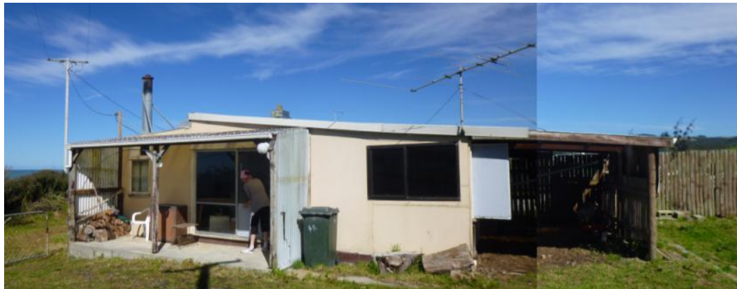
Figure 163. North Elevation of the crib, LK March 2014
