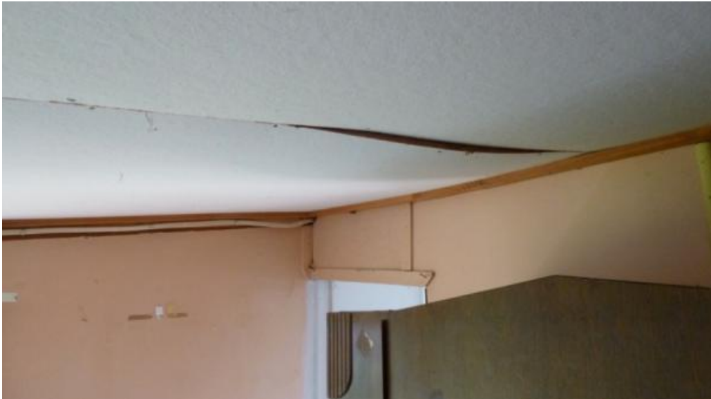
Figure 141. Ceiling in bedroom, GB March 2014
