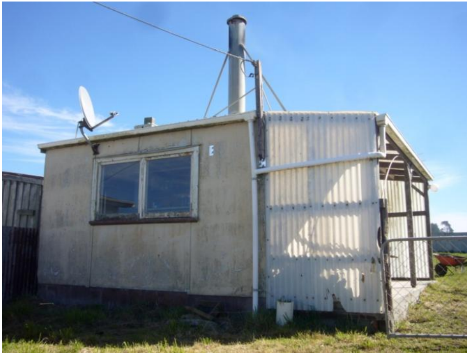
Figure 73. East Elevation of the crib. Photograph: LK March 2014.
