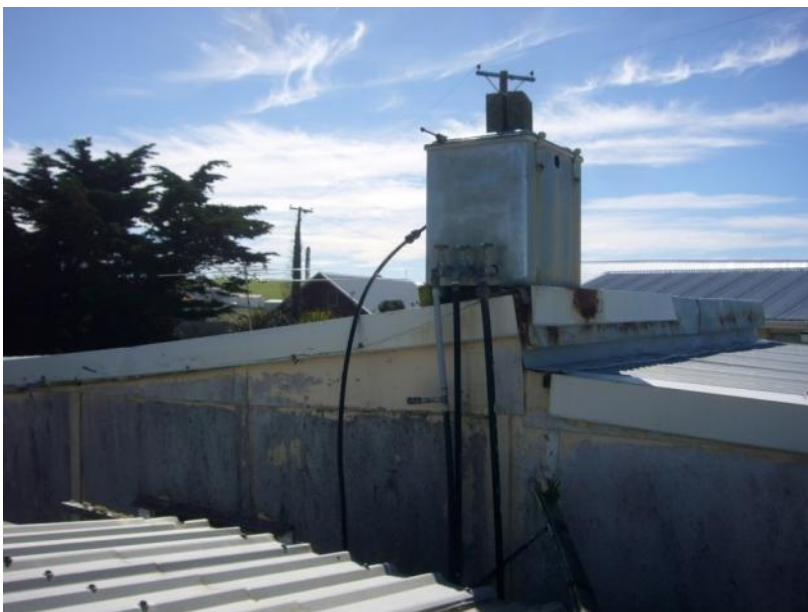
Figure 100. View north showing roofing junctions, GB March 2014
