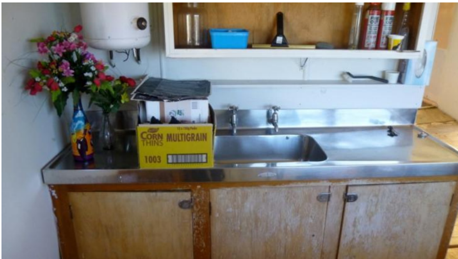
Figure 129. Kitchen cabinetry on west wall of kitchen, LK March 2014
