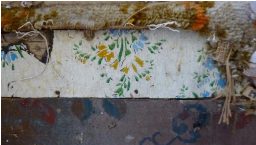
Figure 142. Layered flooring in bedroom, GB March 2014
