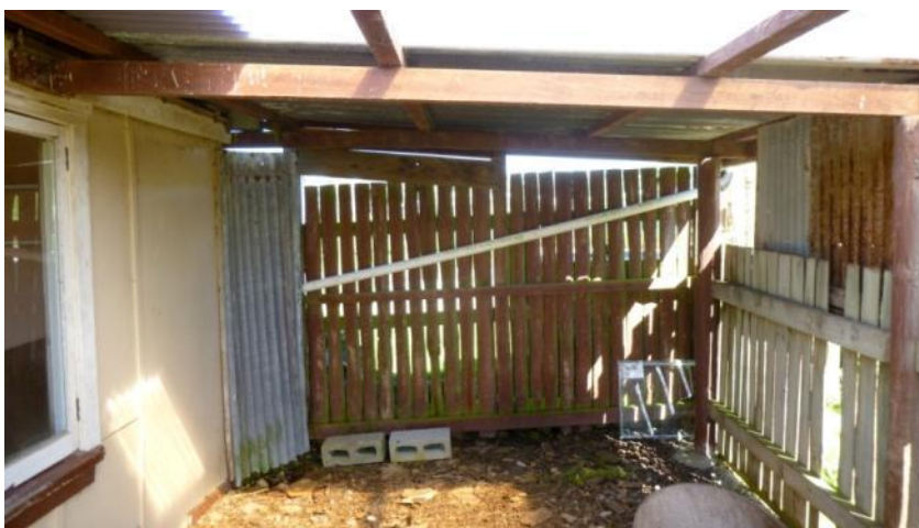
Figure 165. South wall of lean to carport GB March 2014
