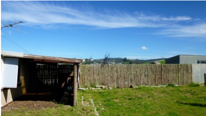
Figure 164. North elevation of lean to carport showing south boundary fence GB March 2014
