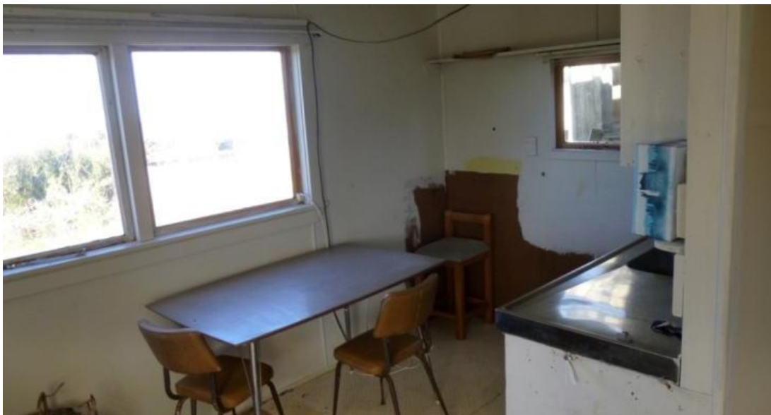
Figure 115. South east corner kitchen area as viewed from doorway into living area, LK March 2014
