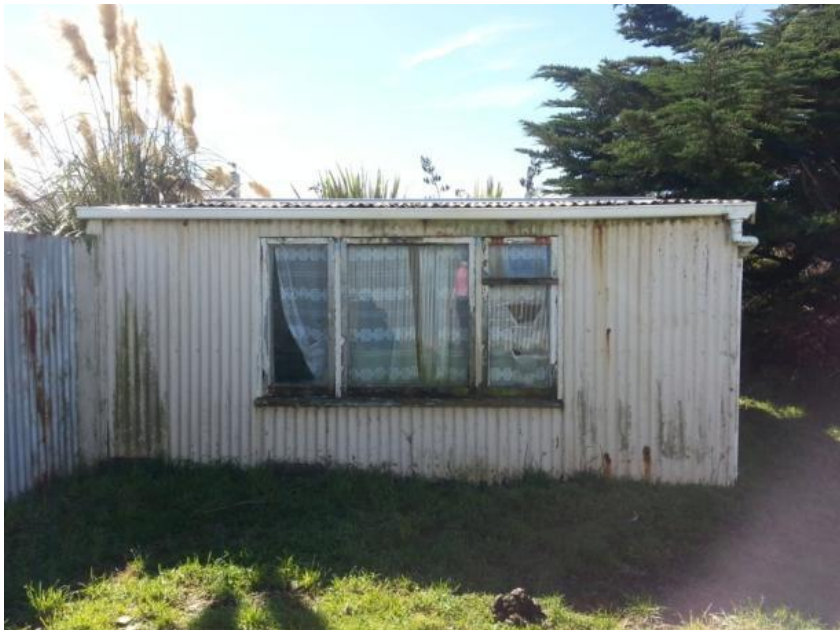
Figure 185. South elevation of the shed, LK March 2014
